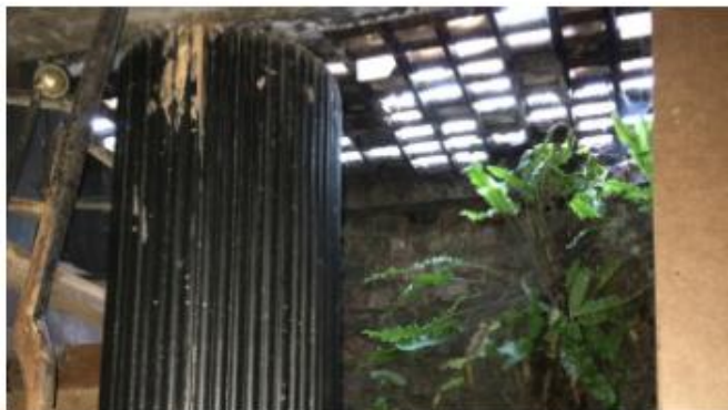
Richardson of Highgate basement area looking up through pavement lights
