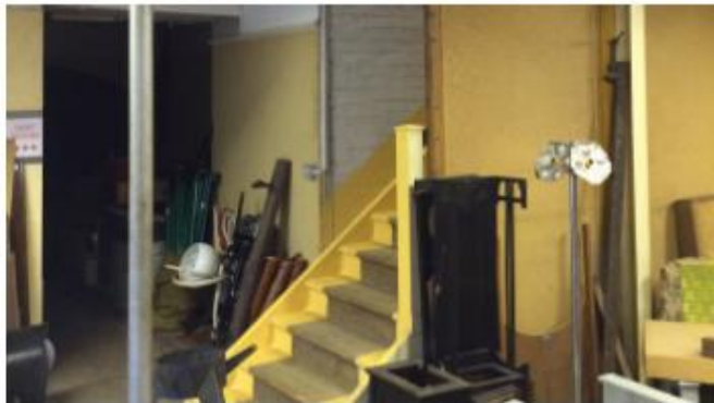
Access down to Richardson of Highgate basement area
