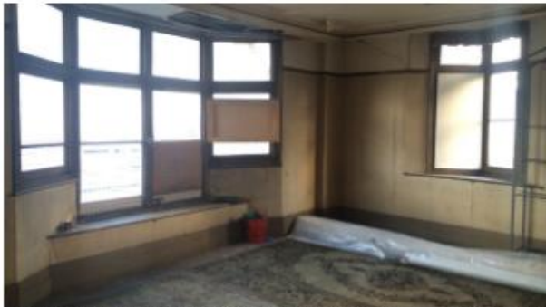
Richardson of Highgate unoccupied shopfloor looking out towards Archway Road through the bay window
