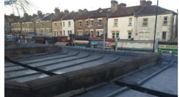
05 View of flat roof above commercial space at ground.
